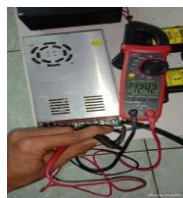
Gambar 8. Pengujian power supply
