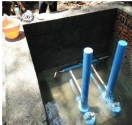
Gambar 2 Pompa hidram (Asmaranto et al, 2017)
